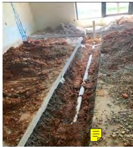
Continue Underground plumbing in area
