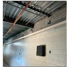
Continue installing new conduit overhead
