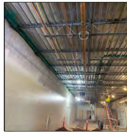
Continue installing refrigerant piping overhead
